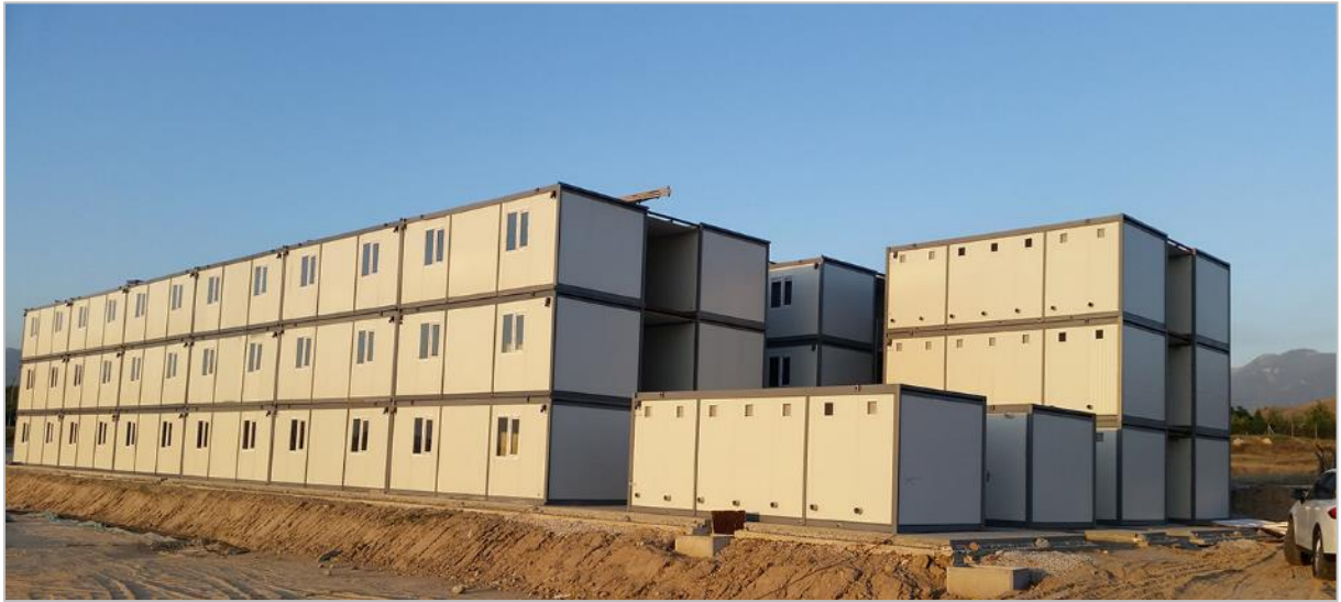
Photo 9- Modular Labor Accommodation Camps from containers
